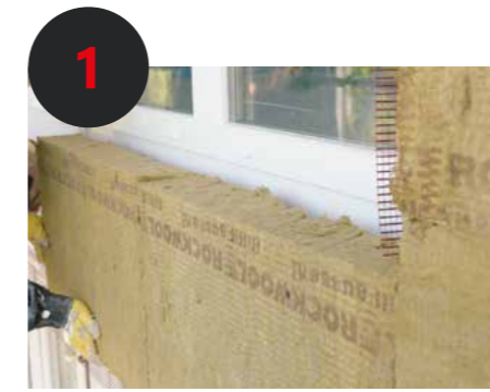
1 Application of insulation panels to the facade
