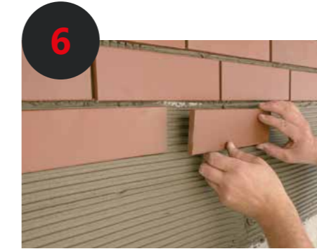
6 Setting the slip in the adhesive
