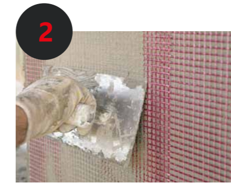
2 Installation of a reinforcement layer
